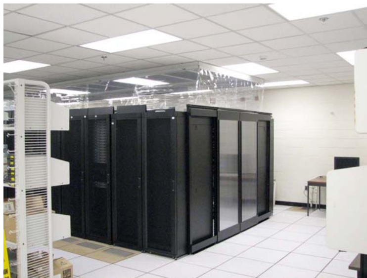
Installation of Hot Isle Containment
